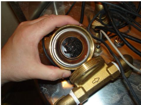
In the interior of the pump, the impeller wheel will now be visible.
